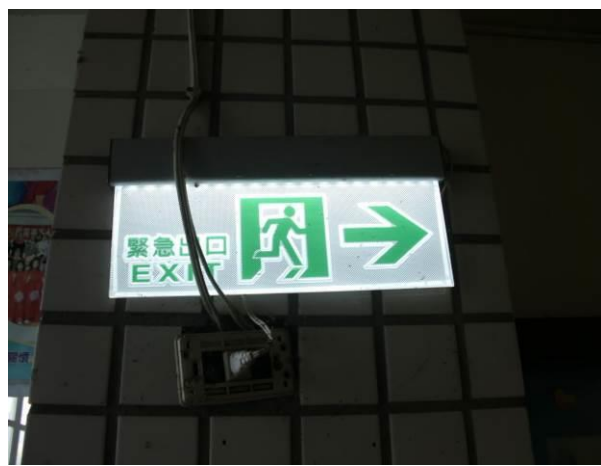
更換省電 LED 燈－逃生指示燈
